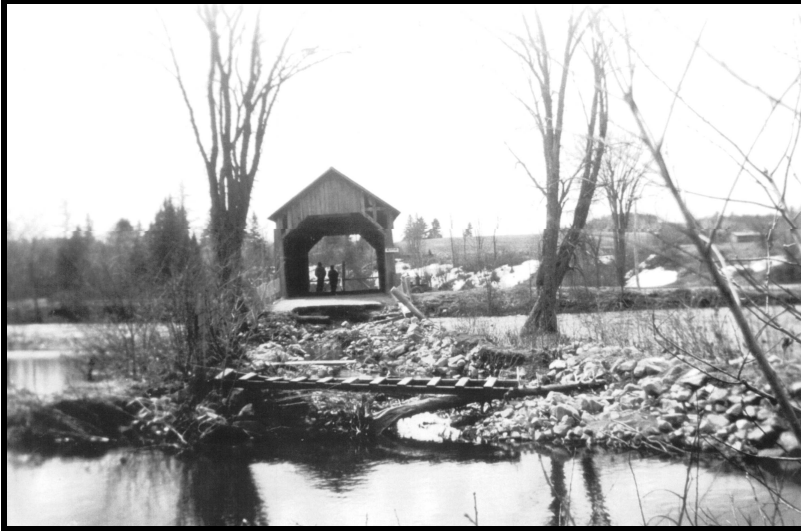
Damage caused by Keswick River flood, Zealand Covered Bridge, 1950.
