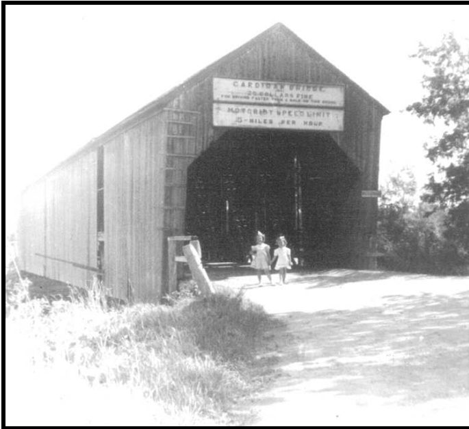
Burt's Corner bridge "Cardigan Bridge", washed out in 1970.
